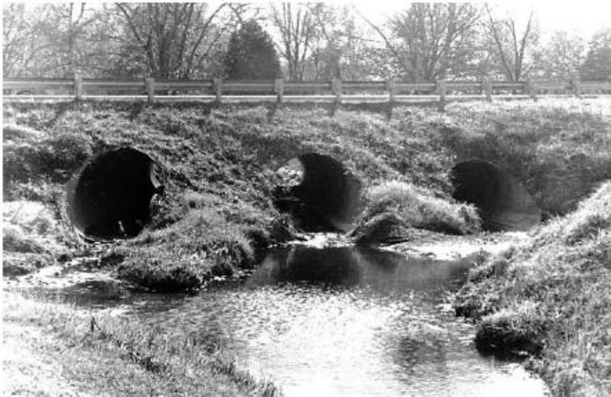
Figure 8 Corrugated Metal Arch Culvert
