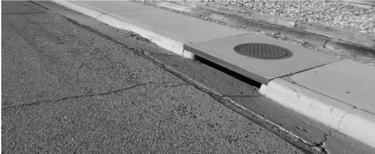
Figure 7 Curb and Gutter
